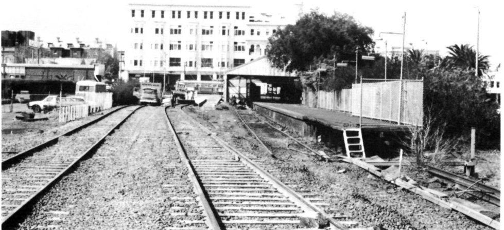
The LRV line runs through the former goods yard at St Kilda Station to join Fitzroy Street at Grey Street. The 5ft 3in gauge station is on the right and the former 5ft 3in gauge Victorian Railways electric tramway from Brighton terminated to the right of the station building.
