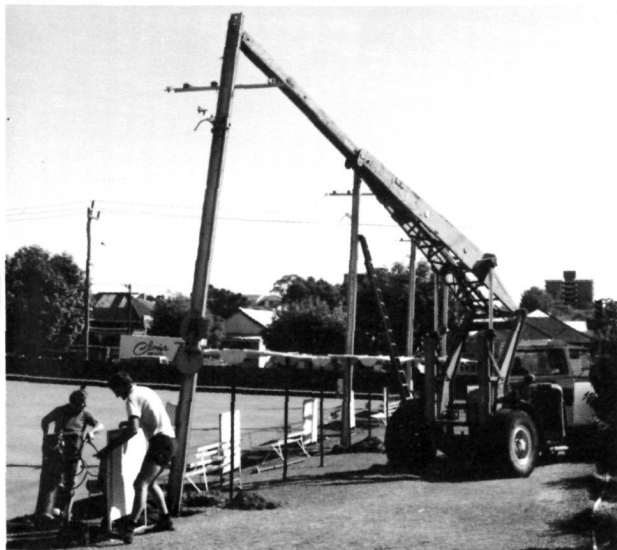
Royal Park Bowling Club, 13 April 1987. Reg Francis and Duncan McVicar move clear as the crane takes the weight of a tram rail pole. Four poles were 'felled' at each end of the three bowling greens.
