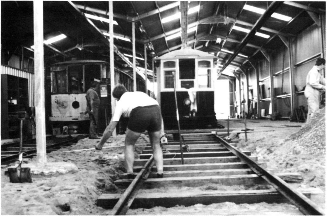
Tracklaying in the carbarn extension was well in hand on 19 July 1987, with Martin Grant (far left), Reg Francis, John Shaw and Ron Hood hard at work. Former Fremantle trams 14 (left) and 29 are behind them.
