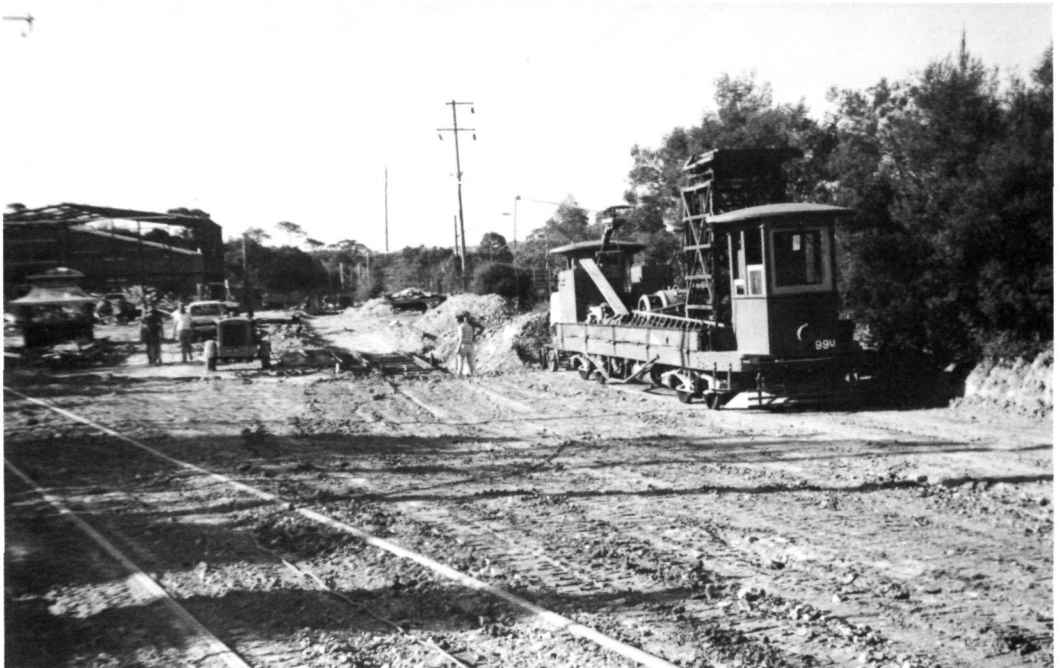
Ballast motor 99U became the first tram on Tramway Avenue at 3.50 pm on 19 September 1987.
