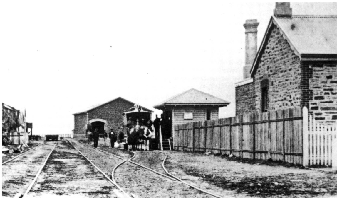
Victor Harbor station circa 1880. A saloon tramcar is about to leave for Goolwa. The stone goods shed, which still stands at Victor Harbor and houses the present tramcar fleet, appears beyond the horse tram. Note how the space between the rail is built up to provide a footing for the horses.
