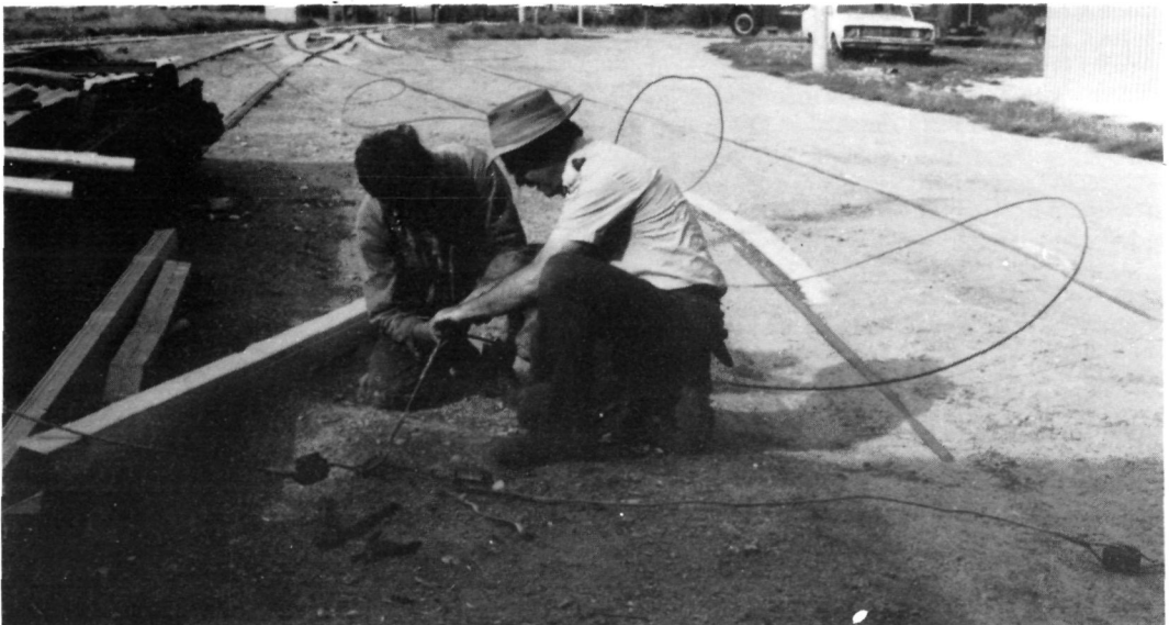
Tony Smith and John Lambert splicing the pull-off for the No. 1 road trolley wire.
