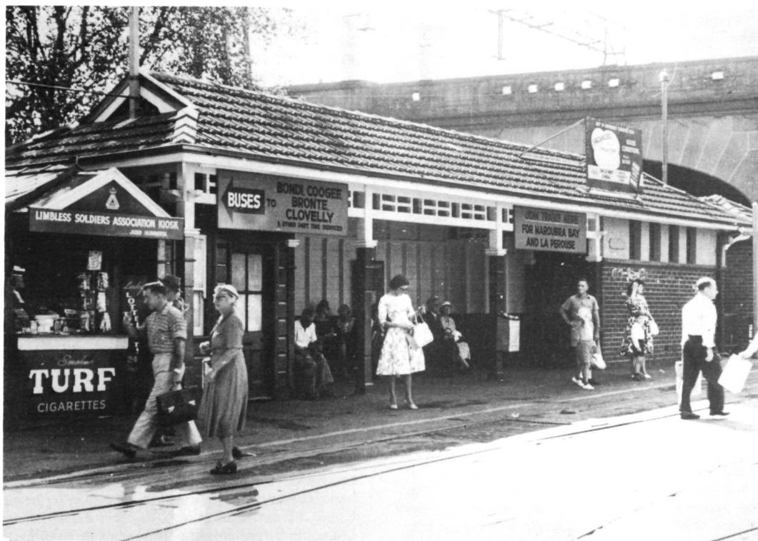
The recently demolished waiting shed in Eddy Avenue, Sydney. This view was taken in January 1961, a few weeks before the trams ceased running.
