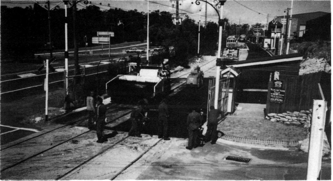
Sutherland Shire Council's paving contractors complete the tar sealing of Tramway Avenue on 22 August. W2 class 392, in the background, was used to run the grooves in the hotmix surface.
