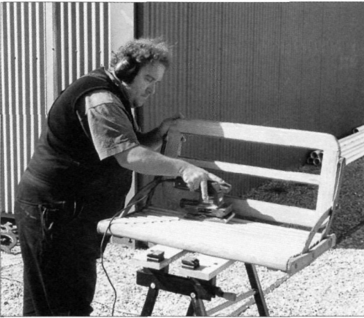
John Stone sands a seat for Perth E class 66 on 17 July, and Roy Winslow re-assembles it – one down, 27 to go ... Michael Stukely
