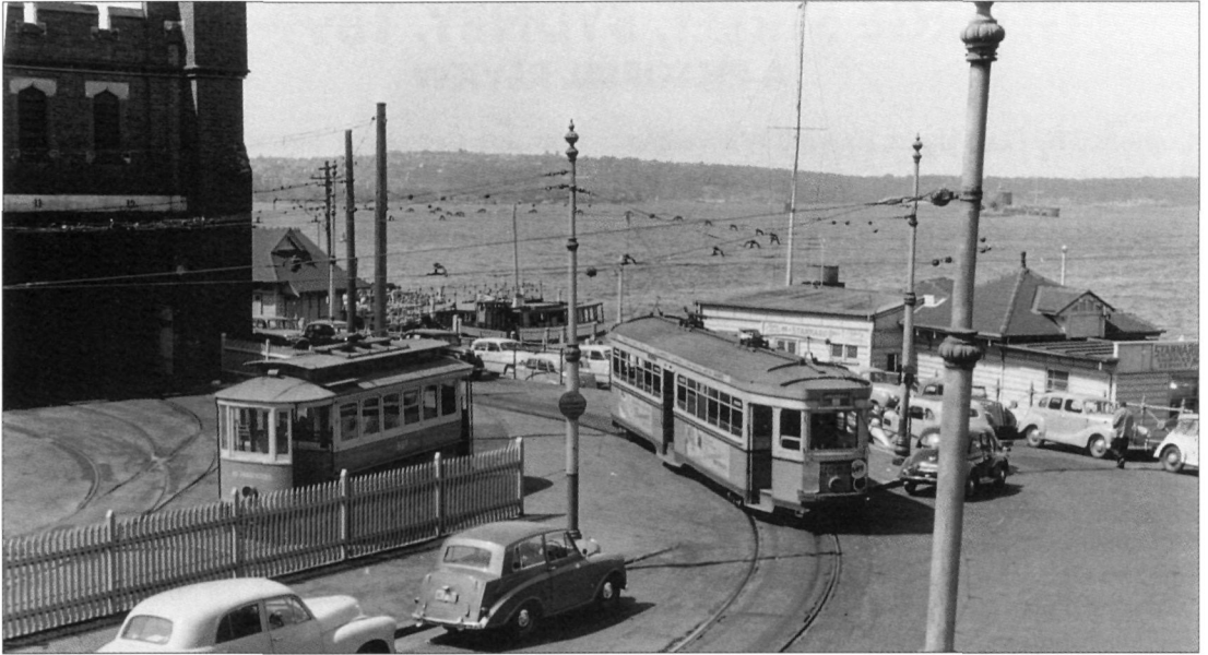
R1 car 2052 is passing the south-eastern corner of Fort Macquarie depot at the start of a run to Annandale in 1955. At left is breakdown car 56s, which was attached to the depot from 1909 until it closed in October 1955. After use as an advertising car (see the back page) and on tours, this car was bought by Mr Norm Boxall and after almost 40 years of outside storage is now at the Sydney Tramway Museum. Noel Reed
