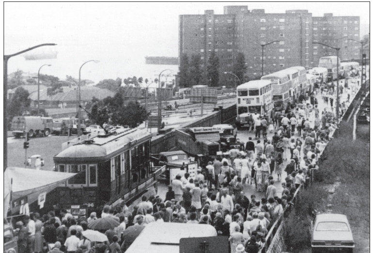
K 1296 and road vehicles on the former tramway right-of-way on the northern approach to the bridge on 21 March 1982.
