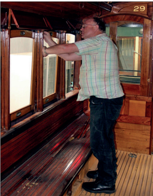
Ian Hanson re-installed the windows in C 29 on 13 April.
