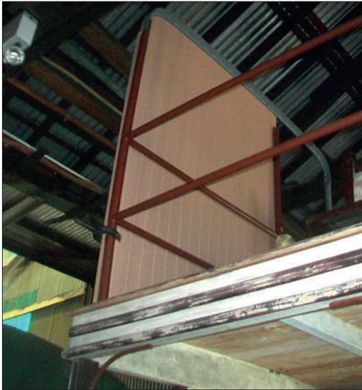
A weather protection board in place on the top deck of the double-deck car.
