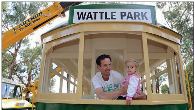
Former SW6 861 installed at Wattle Park.
