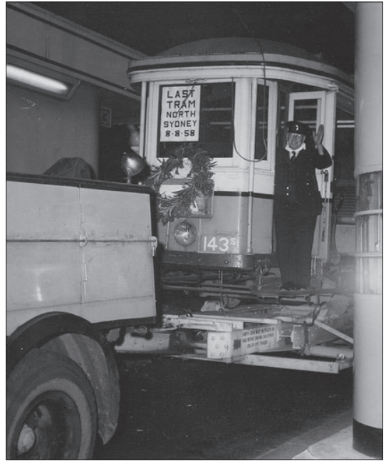
The last tram to leave the North Sydney system, O breakdown car 143s passes through the Sydney Harbour Bridge toll booths on 7 August 1958 behind AEC Matador CT.073. This was the last time the Lizard was used. R.I. Merchant collection
