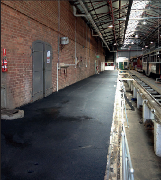
The resurfaced walkway beside road one at the depot.
