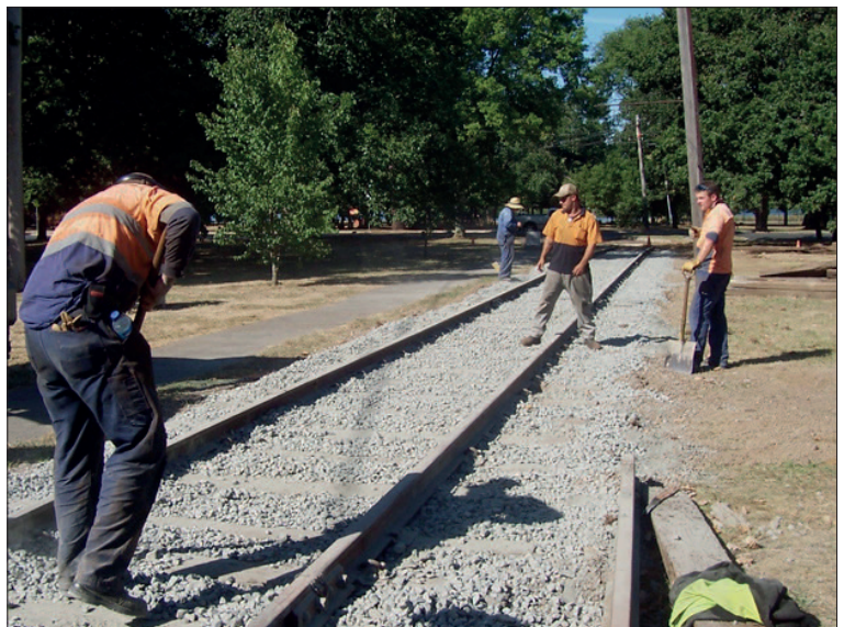
Completing the ballasting on 20 February.
