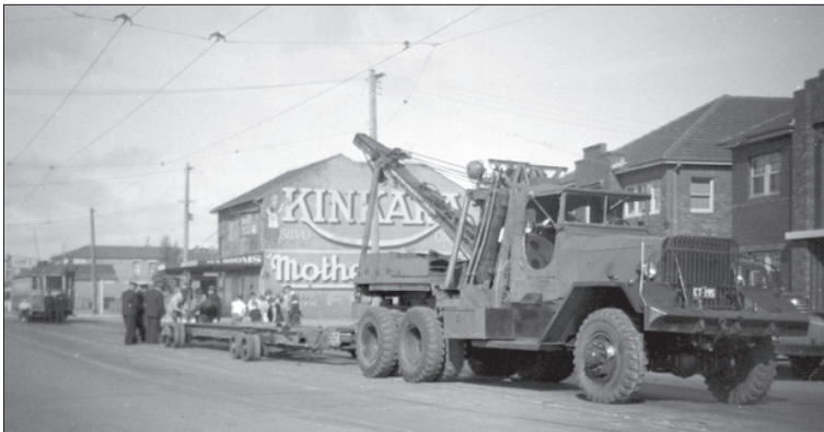
The Kenworth was used to return trams from the Rockdale to Brighton-le-Sands line to Randwick Workshops after the line's closure in 1949. The Lizard trailer is being prepared to load L/P class car 220 in the background. J.W. Burgess
