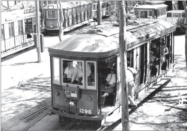
K 1296 inaugurates electric operation at Loftus as it leaves the Sydney Tramway Museum's old site at 11:00am on the morning of 14 March 1965.
