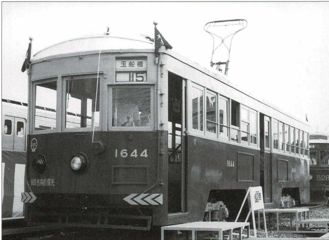
Japanese tramcar practice standardised on front and centre doors and steel-bodied 1644 reflects this design. It also had rear doors when built in 1929.
