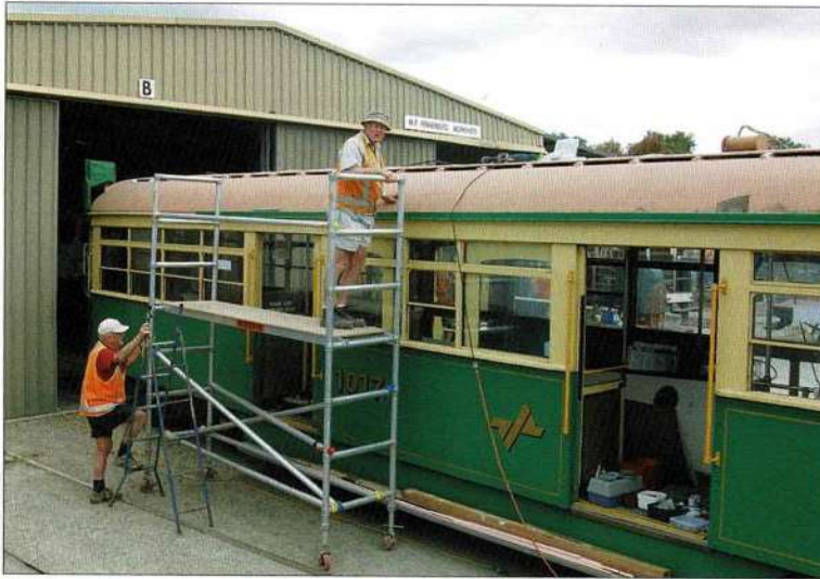
John Davies (left) and Graham Bedells carrying out repairs to the roof of W7 1017 on 20 October, outside the W.P. Pennenburg Workshop.
