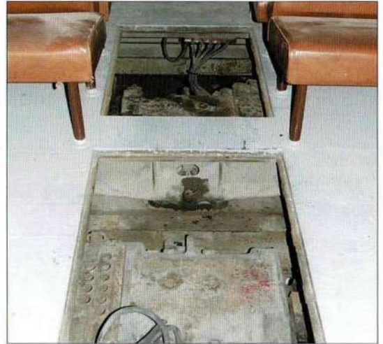
The new trucks for 1013 seen through the car's floor hatches.
