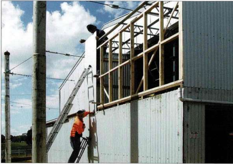
Frank Schroeders and Anthony Smith clad the extension to 3 Road. Jacqui Smith
