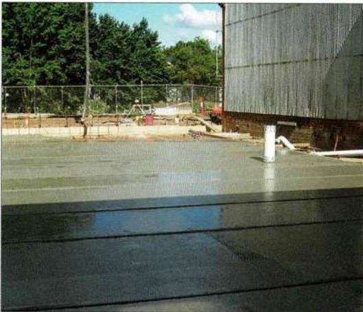
The freshly laid concrete slab for the depot extension. Bendigo Tramways
