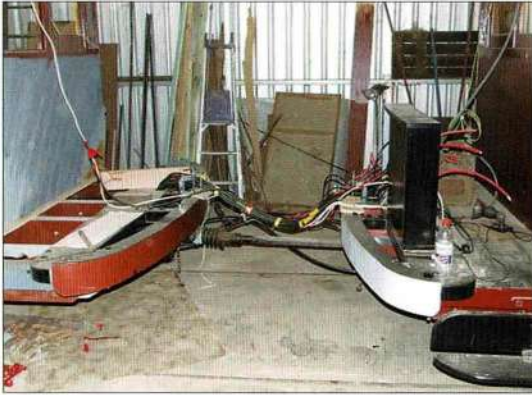
The spring-compensating towbar installed between 14 and 15. Most of the temporary resistor banks that were previously on the cab floor of No. 15 have been relocated beneath the floors of these trams.
