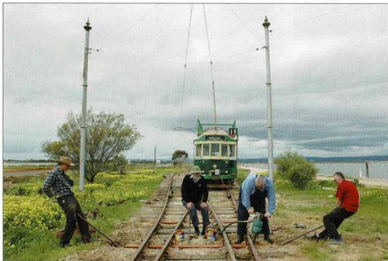
Mark Jordan, Jack Pennack, Kym Smith and Charlie Rodgers hard at work replacing point timbers at Mangrove Loop on 11 September 2010.
