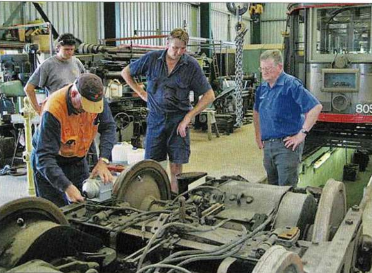
Bill Parkinson takes a 'megger' reading from a motor in one of 805's bogies. The results were quite satisfactory and the car's electricals were found to be in very good condition. Dave Rockell, the Powerhouse Museum's Acting Manager, Conservation, (centre) is keeping an eye on the work being carried out.
