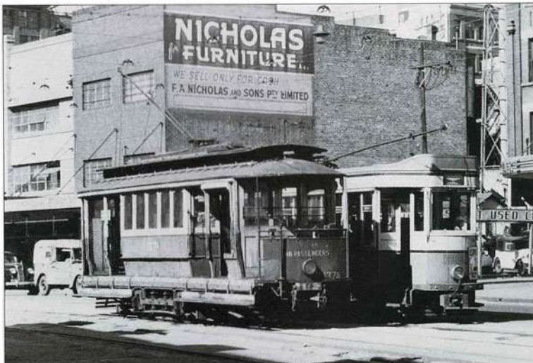
D scrubber 137s, still with an open front, is passed by P 1689 during track relaying work in Broadway in 1950.
