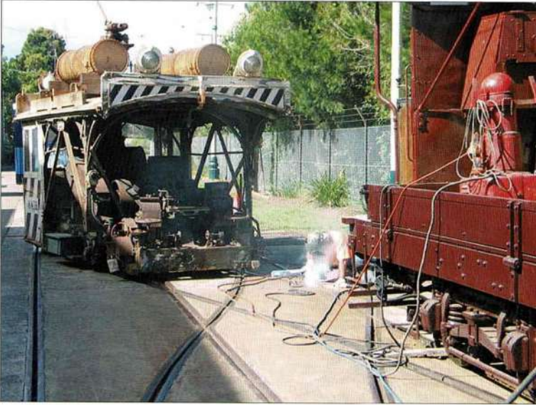
Danny Adamopoulos welds up a worn frog on our scissors crossover. Grinder 3 is standing by, ready to finish the job.
