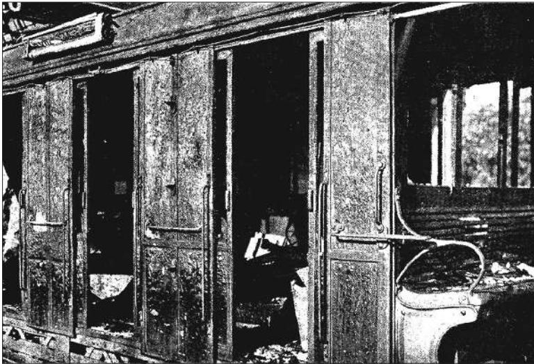
An exterior view of the fire damage to O car 855 in Rozelle Depot.
