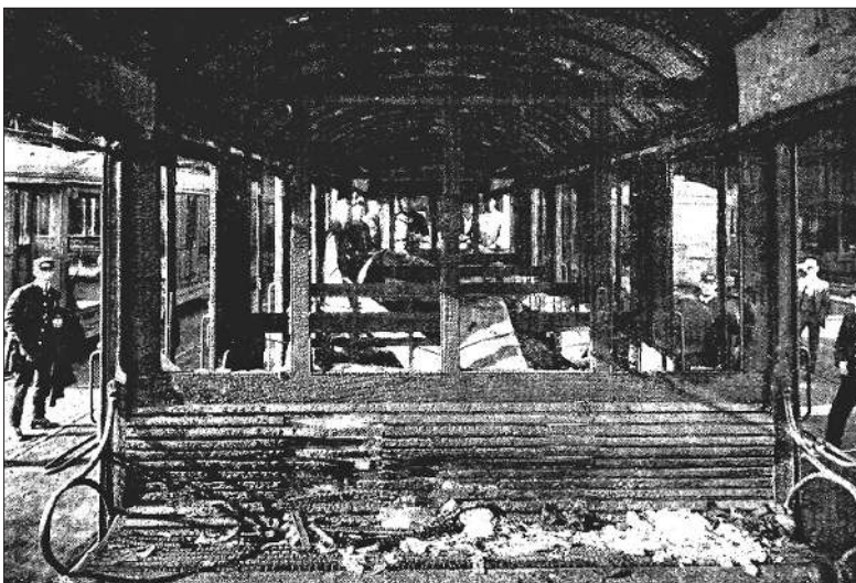
A view inside the fire damaged O car 855 at Rozelle Depot.
