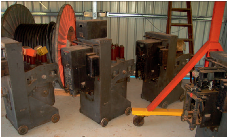
11kV switchgear components being moved to the new substation.
