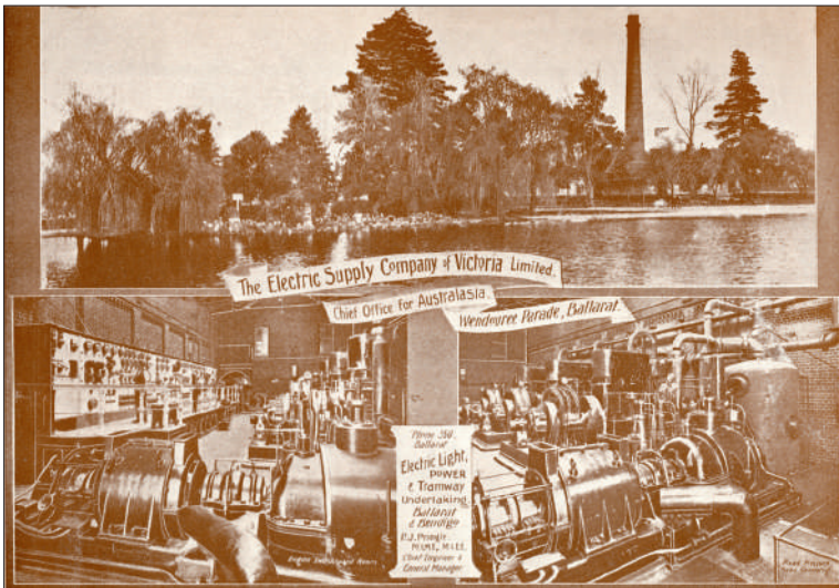
The View Point powerhouse, Ballarat, viewed from across Lake Wendouree. The lower left portion of this card illustrates the engine switchboard room and the lower right shows the fixed pressure turbo generator.
