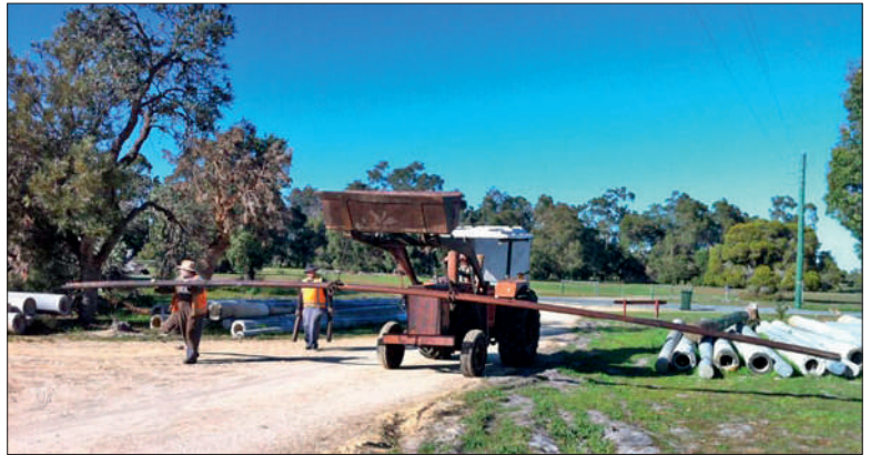
A length of rail is carted from the rail compound to be installed on the new truck storage road on 21 July. Some of the spun concrete poles obtained in 2011 can be seen at right.
