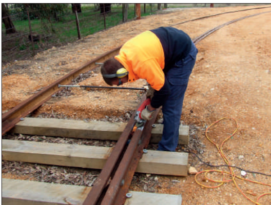
Alastair Reither grinds and surfaces one of the welds to smooth it prior to test running.
