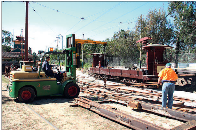
Bill Parkinson uses the fork lift to move rails on 8 September.
