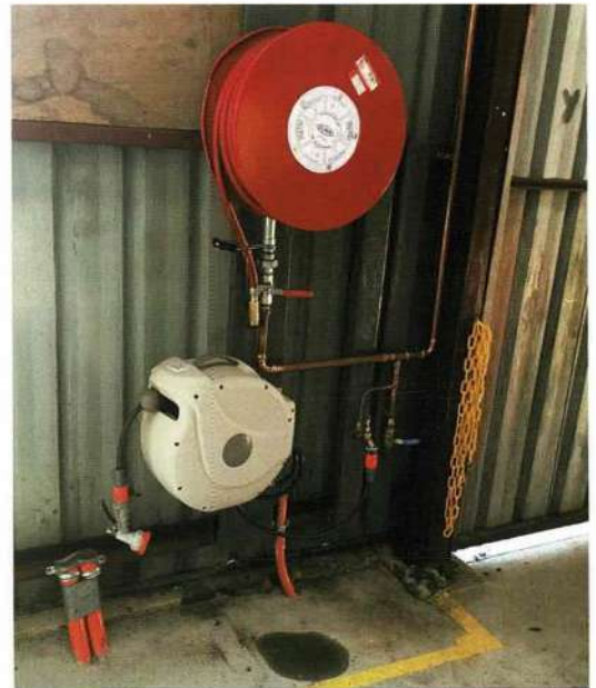
The new fire hose reel and accessories.
