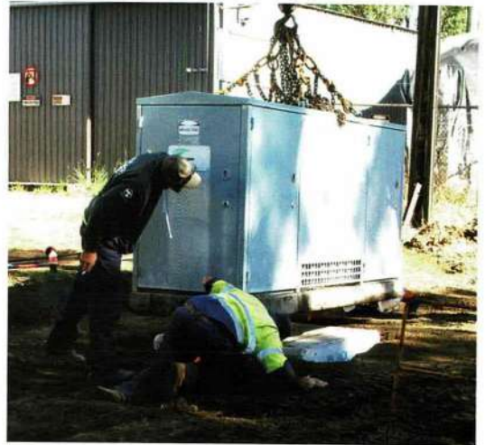
The new transformer is lowered into position.
