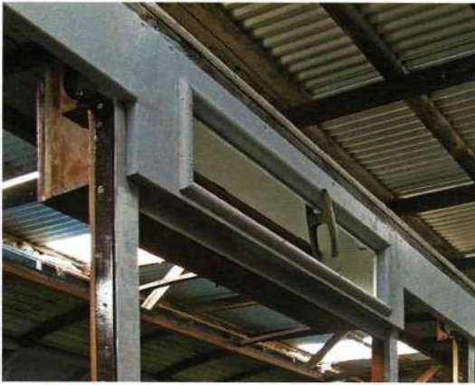
'D' mould trim being fitted to the side destination box fascia of 792. Anthony Smith
