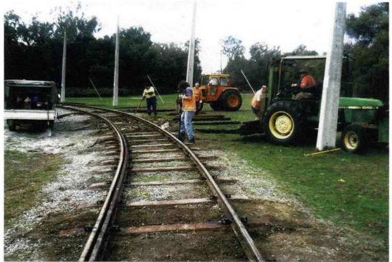
On 14 July, work has progressed to the centre of Farmgate Curve. Nick Tsiaglis (left) clears the remains of a timber sleeper, while Michael Stukely shovel-packs a newly-installed steel sleeper; Terry Young and Trevor Dennhardt are assisting as Roy Daley collects the old timber sleepers with the fork-lift for disposal.
