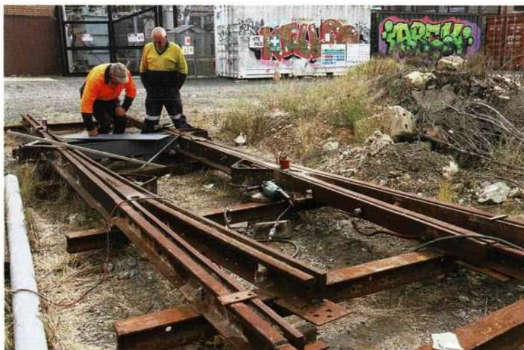
Michael Giddey and Ian Saxon inspect the ex-Dockland set of left-hand points in the northern yard. Martin Pinches
