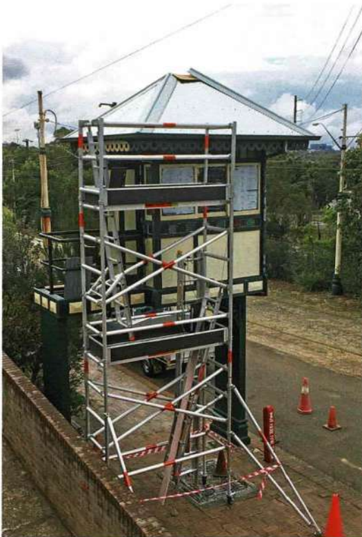
The Liverpool Street Signal Box undergoing its refurbishment. Here the roofing iron is being replaced, 18 September 2018.
