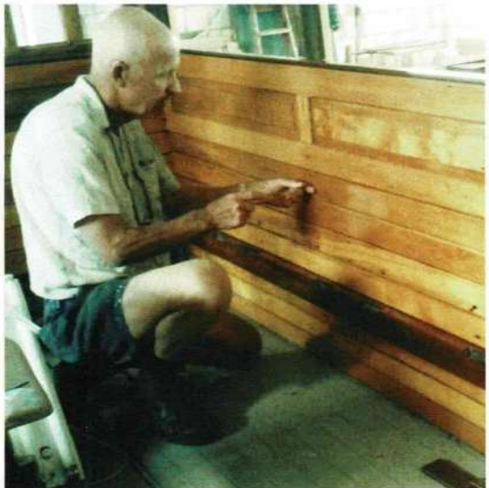
Rob Hodge refitting Huon Pine interior side panels. Note the Huon Pine original panels. John Binns
