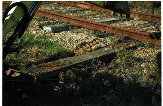
Photos show how sleepers adjacent to the old loop are removed and replaced using an excavator. Nic Benn
