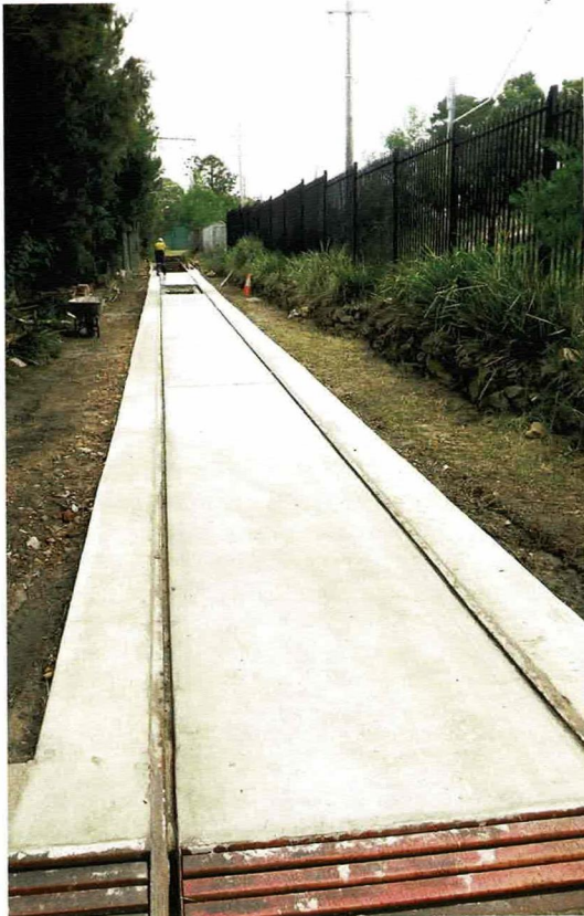
Completing this stretch of concreted track has enabled traffic cars to shunt via the depot junction instead of using Cross Street. 26 June 2019.
