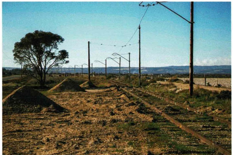
The replacement track adjacent the old loop on 26 June 2019.
