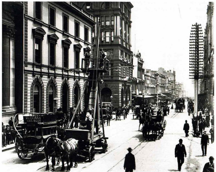
Erecting Mannesmann centre poles in George Street in 1899. State Rail NSW archives
