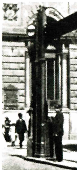
The manually operated signal at the north-west-corner of George Street at King Street. V.C. Solomons Collection
