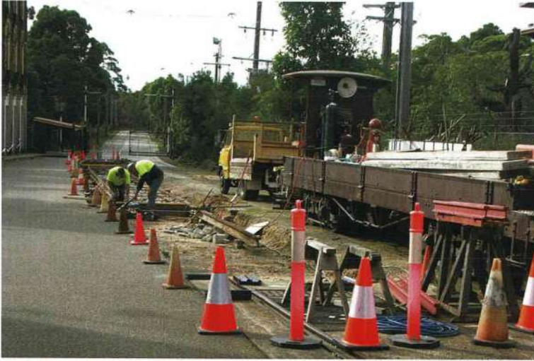
The western track relay work continues in Tramway Avenue on 18 July 2020.
