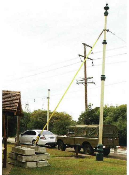
The overhead pole braced in Lakewood Park on 18 July.
