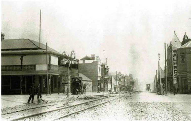
Coburg horse tram rails being removed south of Bell Street in late 1915.
