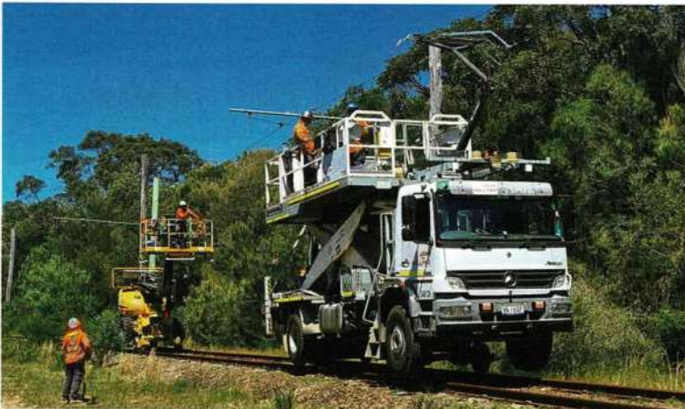
John Holland Rail's two hi-rail work platforms at work Scott Curnow
