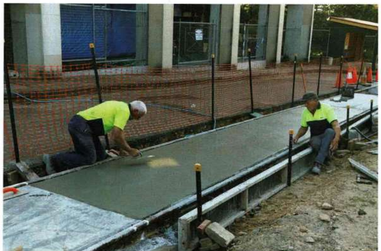
Ian Saxon and Mike Giddey work on smoothing the load received.
