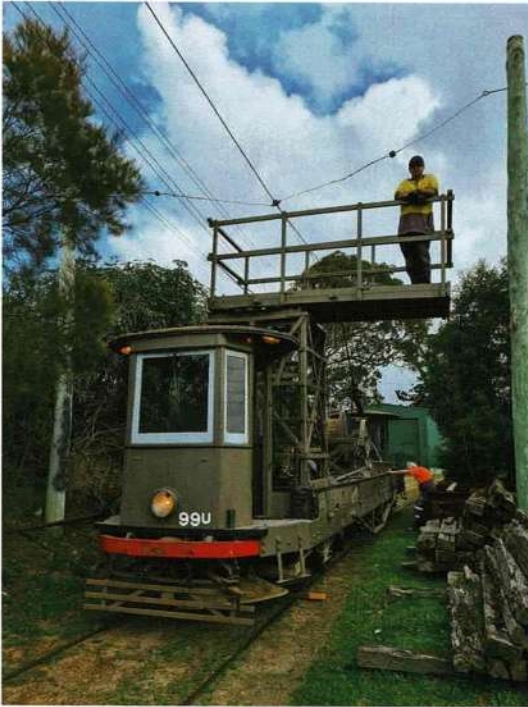
Overhead line car 99u in use on overhead work near the south shed on 19 September. Scott Curnow
