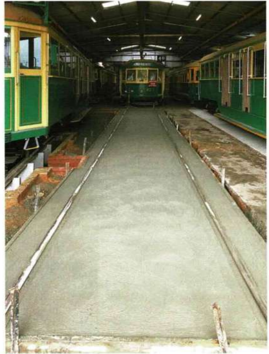
View showing new concrete track on road 4 in the carbarn. Anthony Smith
