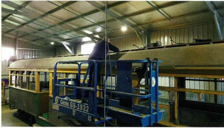
Sim Jenkins works on the roof of 1029 at Bungaree on 21 September 2020.
