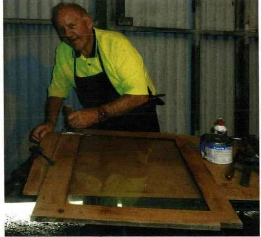
Gavin Casey repairing a window frame on 2 September for return to WGT 130. Lindsay Richardson
