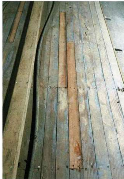
The roof of 1029 showing new timbers that had to be inserted to replace ones that were damaged with holes.
