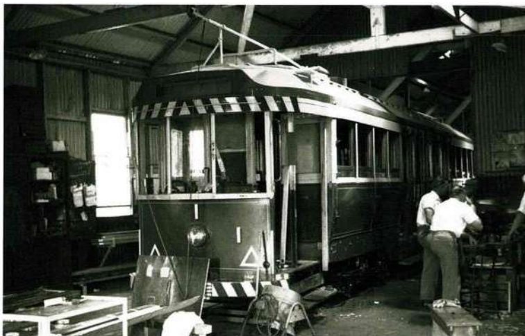
Bendigo No. 1 being converted to become Ballarat 37 (the second one with that number). It shows the front of the tram undergoing modifications to the drivers' door. It arrived from Bendigo on 5 October 1960.
