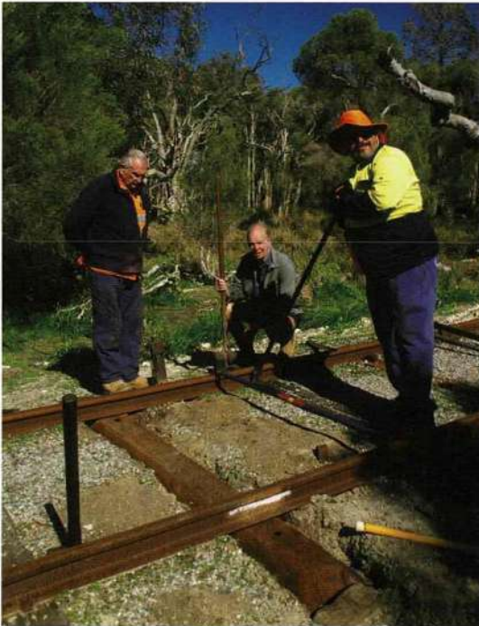
Terry Young (left), Trevor Dennhardt and Nick Tsiaglis checking the track gauge during the installation of steel sleepers on Swamp Straight on 8 August.
