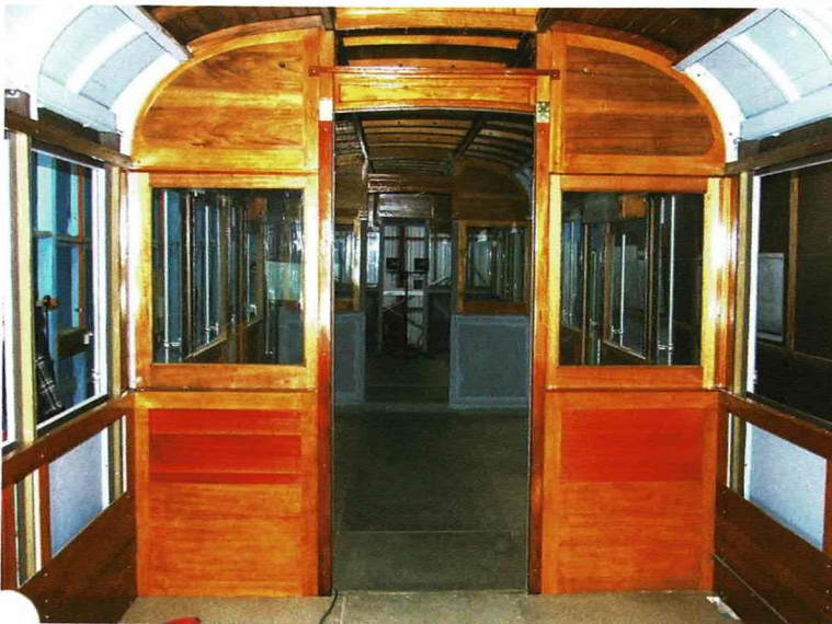
View showing the No. 2 end saloon bulkhead of 792 after the fitting of trim timbers.
