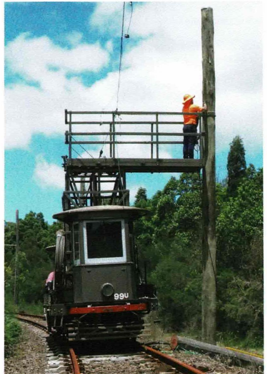
One of the new 11-metre poles being erected on 21 December 2020.
