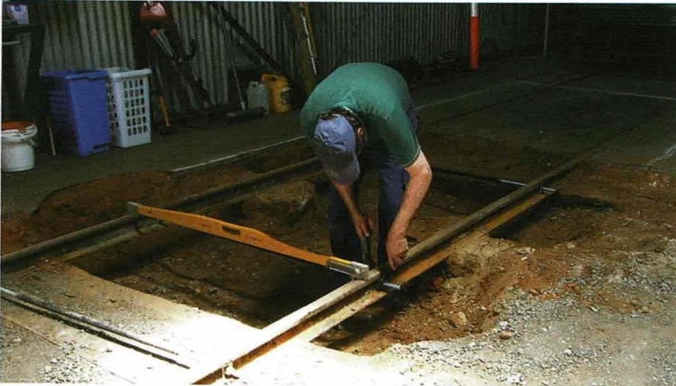
Anthony Smith adjusting tie rods to gauge on No. 3 in the car-barn. Daniel Edwards
