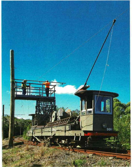
The Sydney Tramway Museum's overhead line car 99u is being used on the Royal National Park line on 9 January 2021 to attach a new overhead bracket arm to one of the two replacement poles required after a November storm brought down a tree which pulled down the overhead wire and two poles either side of it.3
