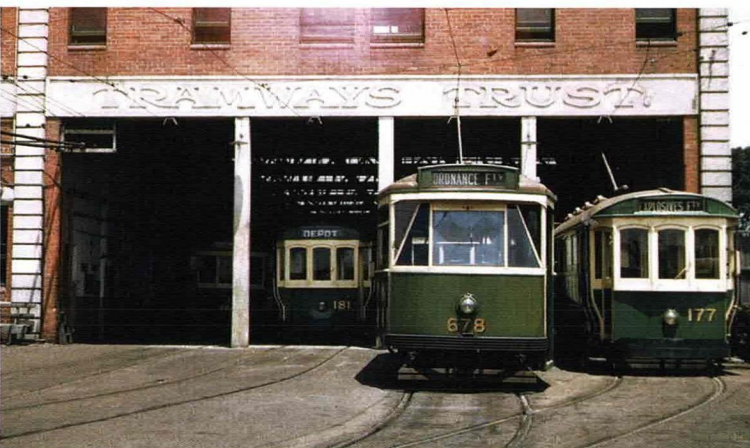
Above, W6 car 1000 in Bourke Street terminus on the opening day of the East Preston line in June 1955.
