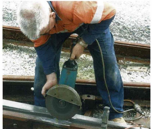
Ray Blackmore hard at it, on 24 March, grinding back a recent weld during his renovation work on the Road 1-2 points on the Oketon Geddes Carbarn fan. Lindsay Richardson
