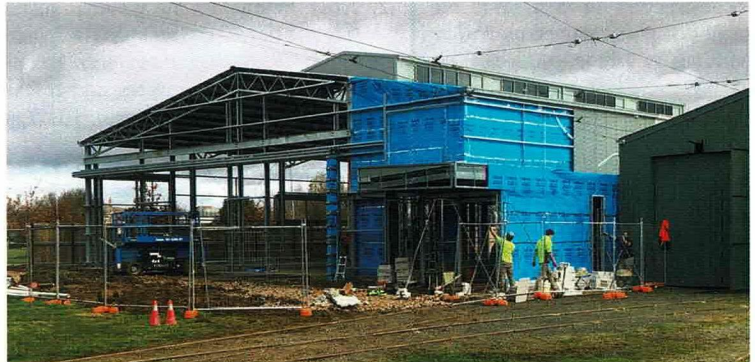
Cladding is underway along with brickwork on 6 July 2021. Warren Doubleday
