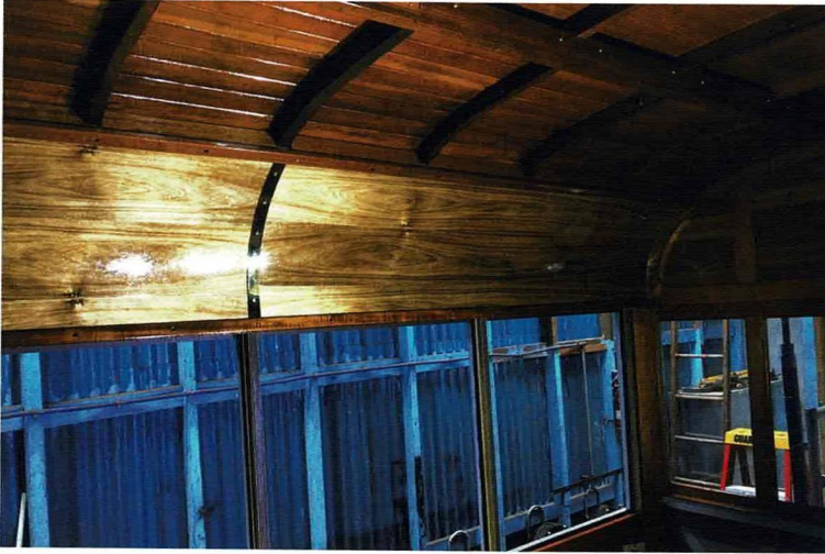
View showing new roof panels and cover strips on 792. Anthony Smith
