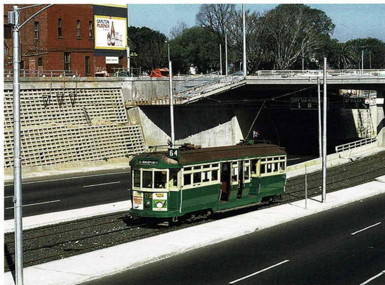
L 103 begins a run along Queens Way on recently-built reserved track, bound for East Brighton in March 1969. Richard Jones
