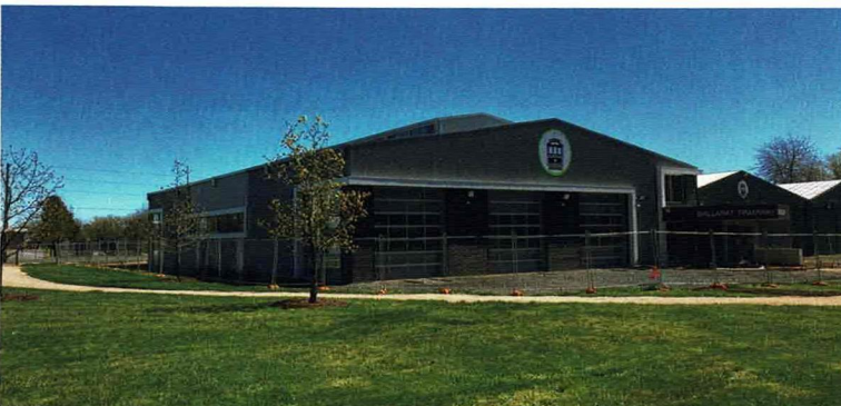
The new building looking north-west on 26 September 2021. Paul Mong
